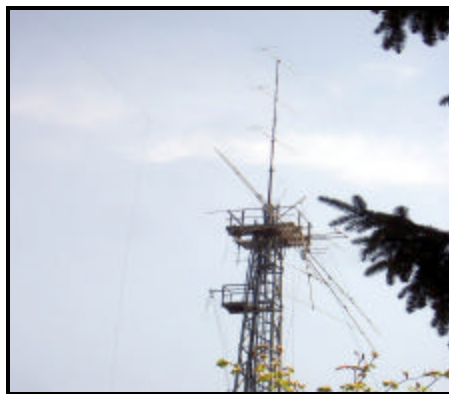
This Guy Was Told He Couldn't Have An Antenna Tower. So He got a permit to drill for Oil and then erected his antennas.
