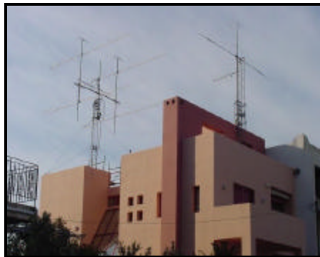
This Operator Was Told He Could Have No Towers In His Yard, On the Roof They Went
